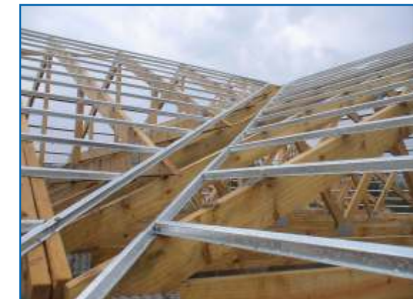
STEEL PURLINS ON TIMBER ROOF
