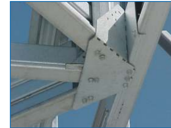
TRUSS TO TRUSS CONNECTIONS
