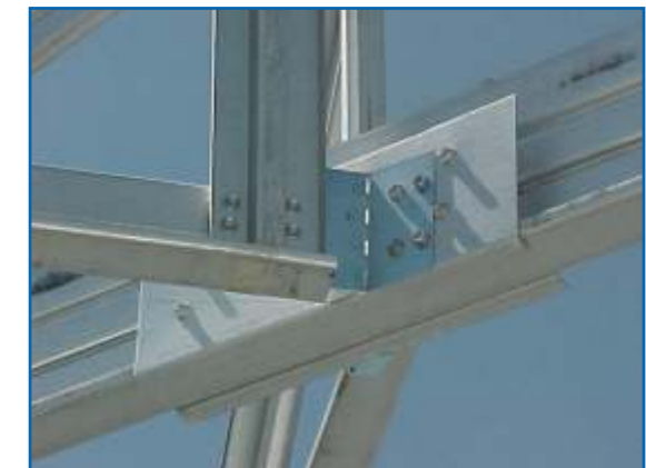
TRUSS TO TRUSS CONNECTIONS
