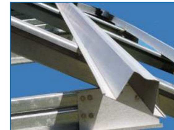
TRUSS TO TRUSS CONNECTIONS
